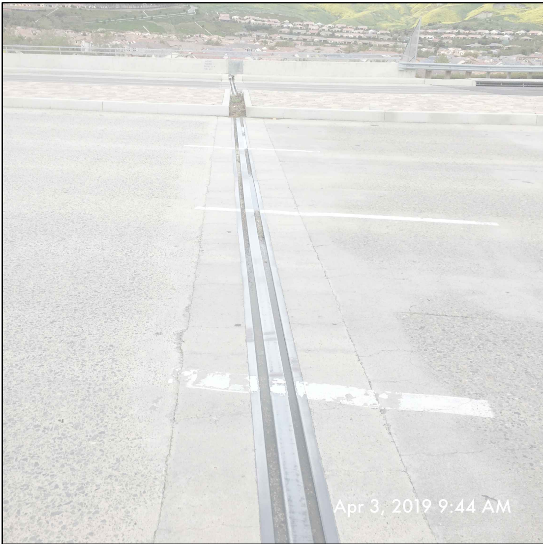
B - EXISTING JOINT SEAL SCALE: NONE
