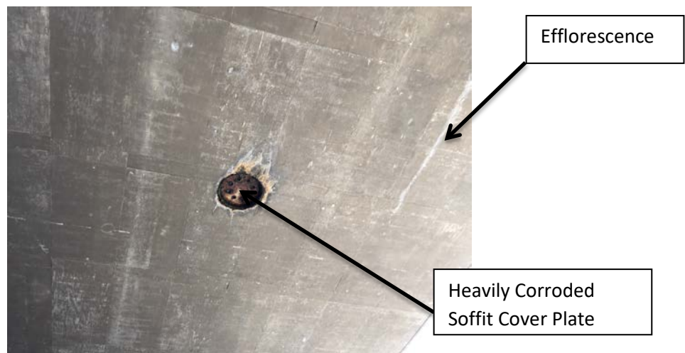
Photo 8: Bridge Soffit
