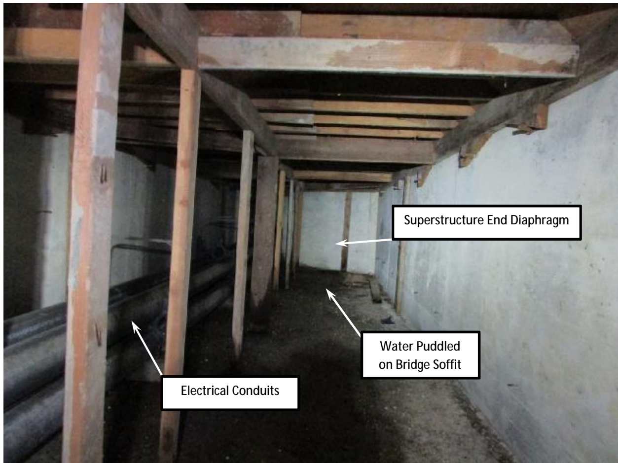
Photo 9: Puddled water by the superstructure diaphragm. There was no indication of water coming from the electrical conduits at this location.
