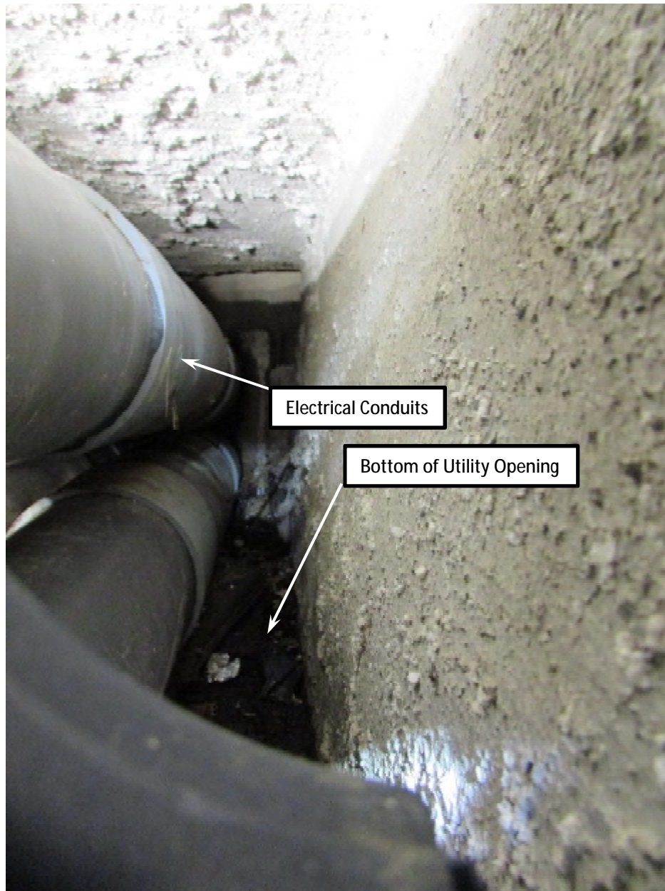
Photo 10: Utility opening through the superstructure diaphragm. The bottom of the utility opening was damp. There was no indication water was leaking from the electrical conduits at this location.
