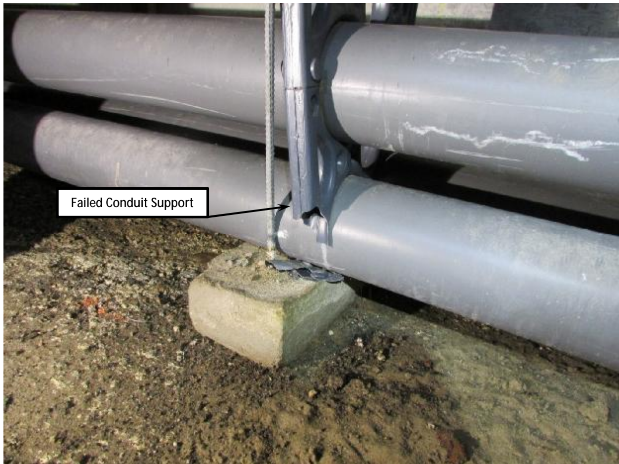
Photo 8: Failed conduit spacer/support likely caused by excessive loads.
