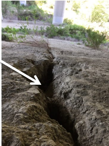
Photo 6: Rutting at abutment
