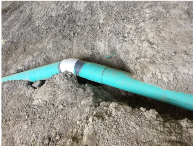
Photo 7: Erosion at abutment weep hole drainage system
