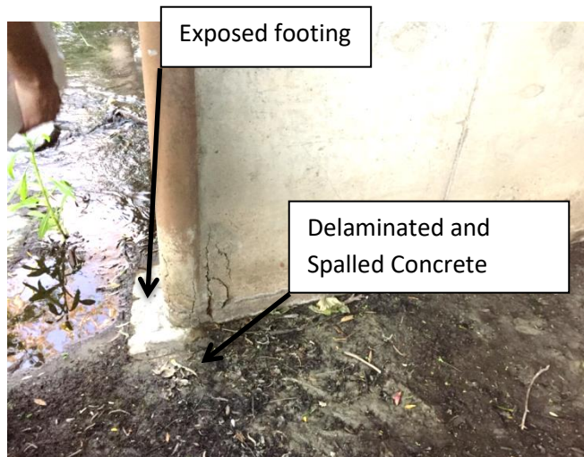
Photo 4: Culvert Wall
