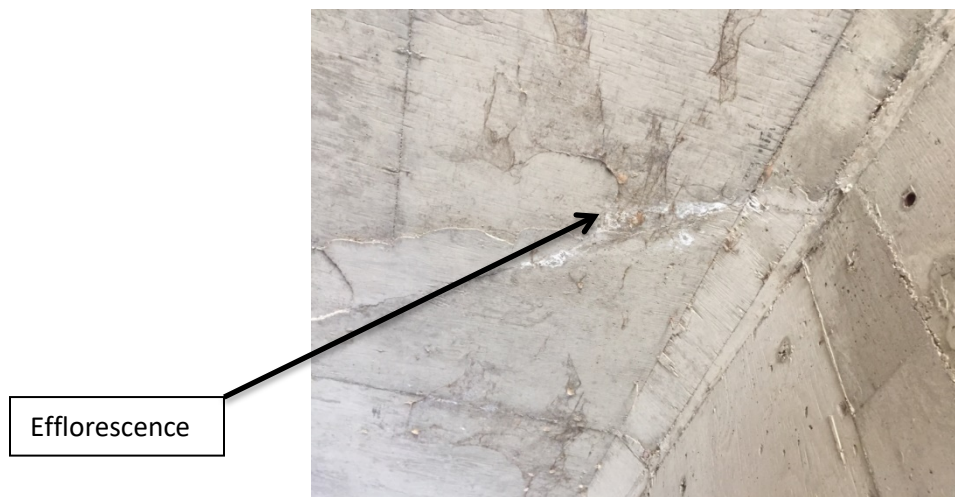
Photo 5: Bridge Soffit
