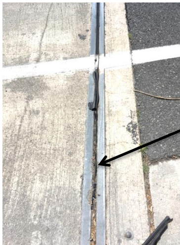
Photo 5: Failed Joint Seal
