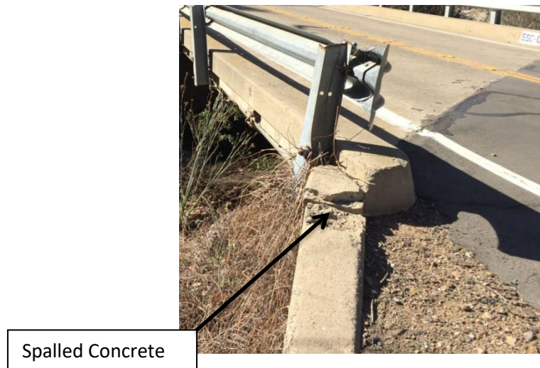
Photo 5: Concrete spalling on wingwall
