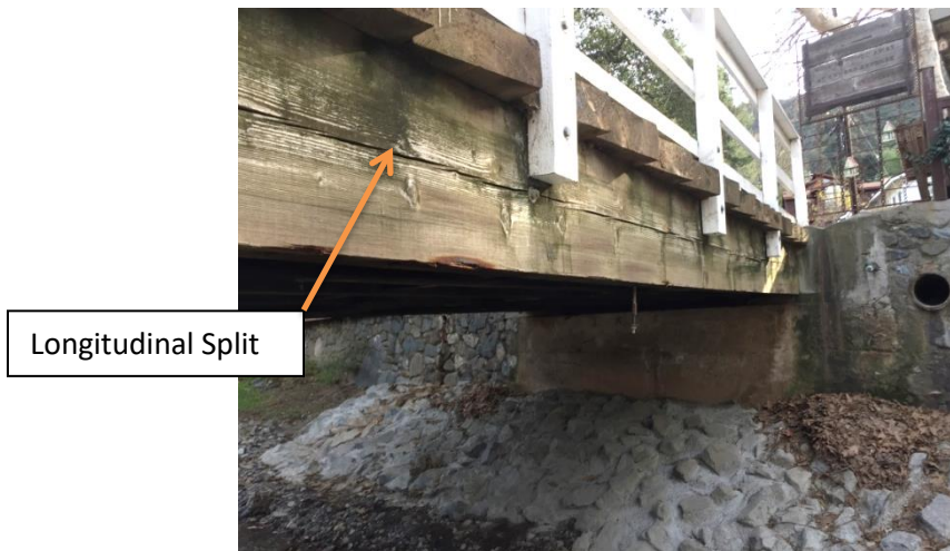
Photo 2: Exterior Stringer with longitudinal split
