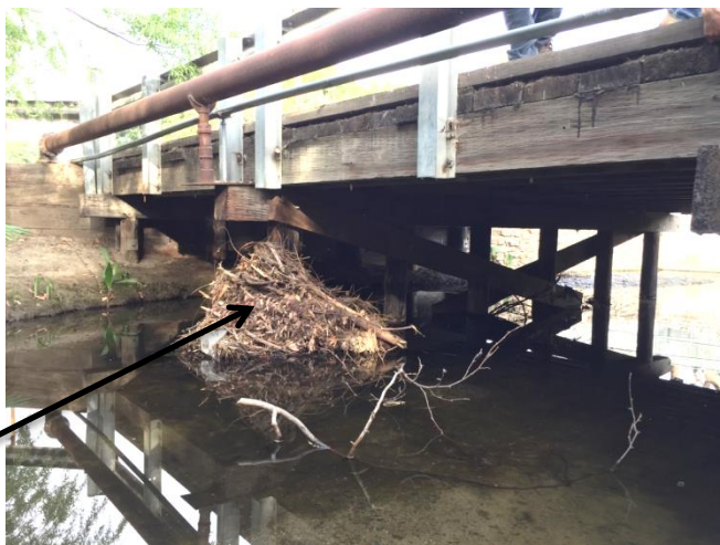
Photo 3: Debris build up on timber columns
