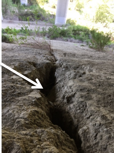
Photo 6: Rutting at abutment
