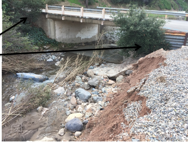
Photo 7: Embankment Erosion
