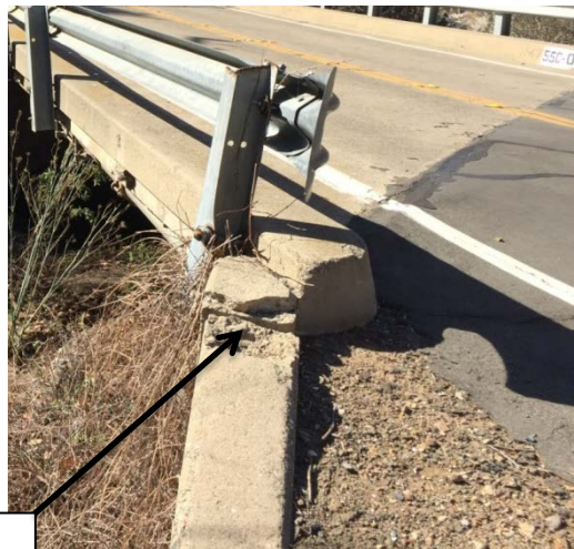
Photo 5: Concrete spalling on wingwall
