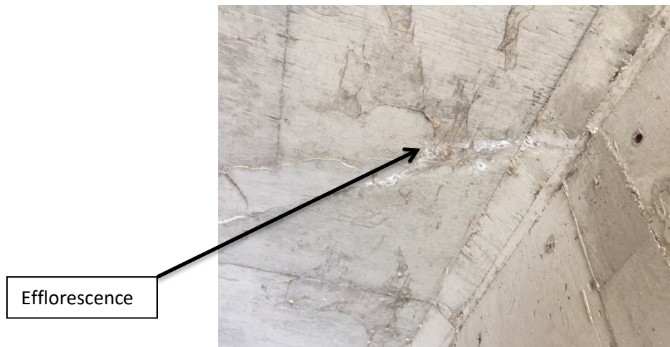
Photo 5: Bridge Soffit
