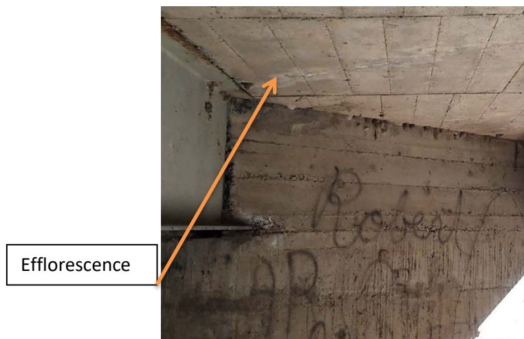
Photo 3: Efflorescence on Bridge Soffit
