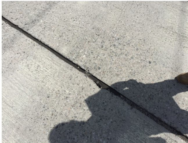
Photo 5: Joint Seal
