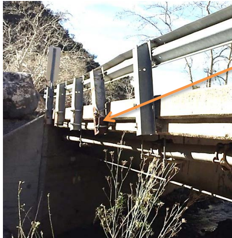
Photo 7: Damaged Metal Post
