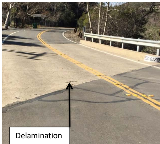
Photo 2: Concrete Delamination on bridge deck
