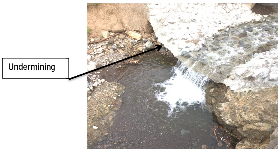
Photo 6: Slope Protection
