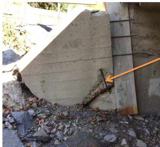
Photo 6: Broken Wingwall
