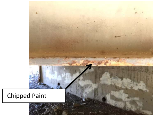
Photo 4: Paint chipping on grinder flange
