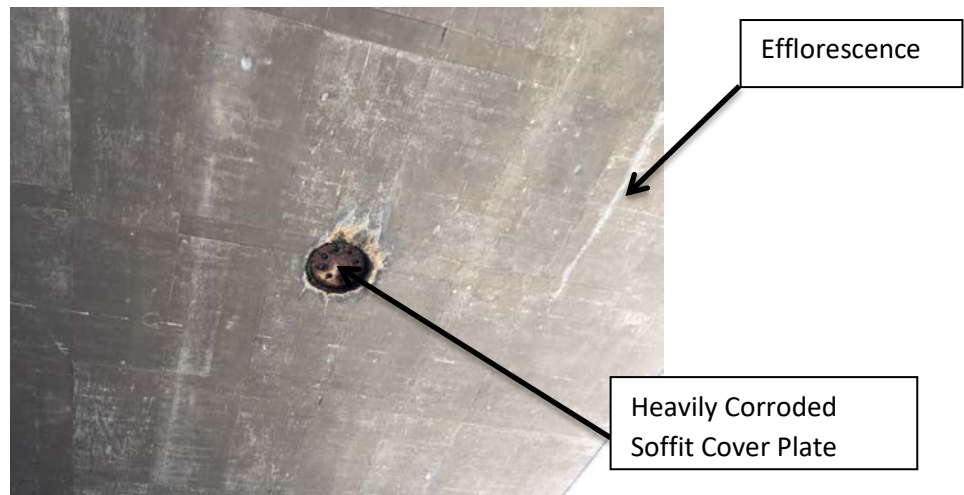
Photo 8: Bridge Soffit
