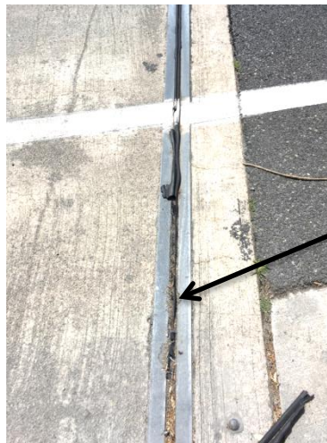
Photo 5: Failed Joint Seal
