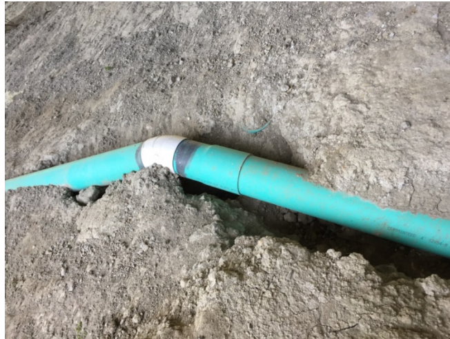
Photo 7: Erosion at abutment weep hole drainage system
