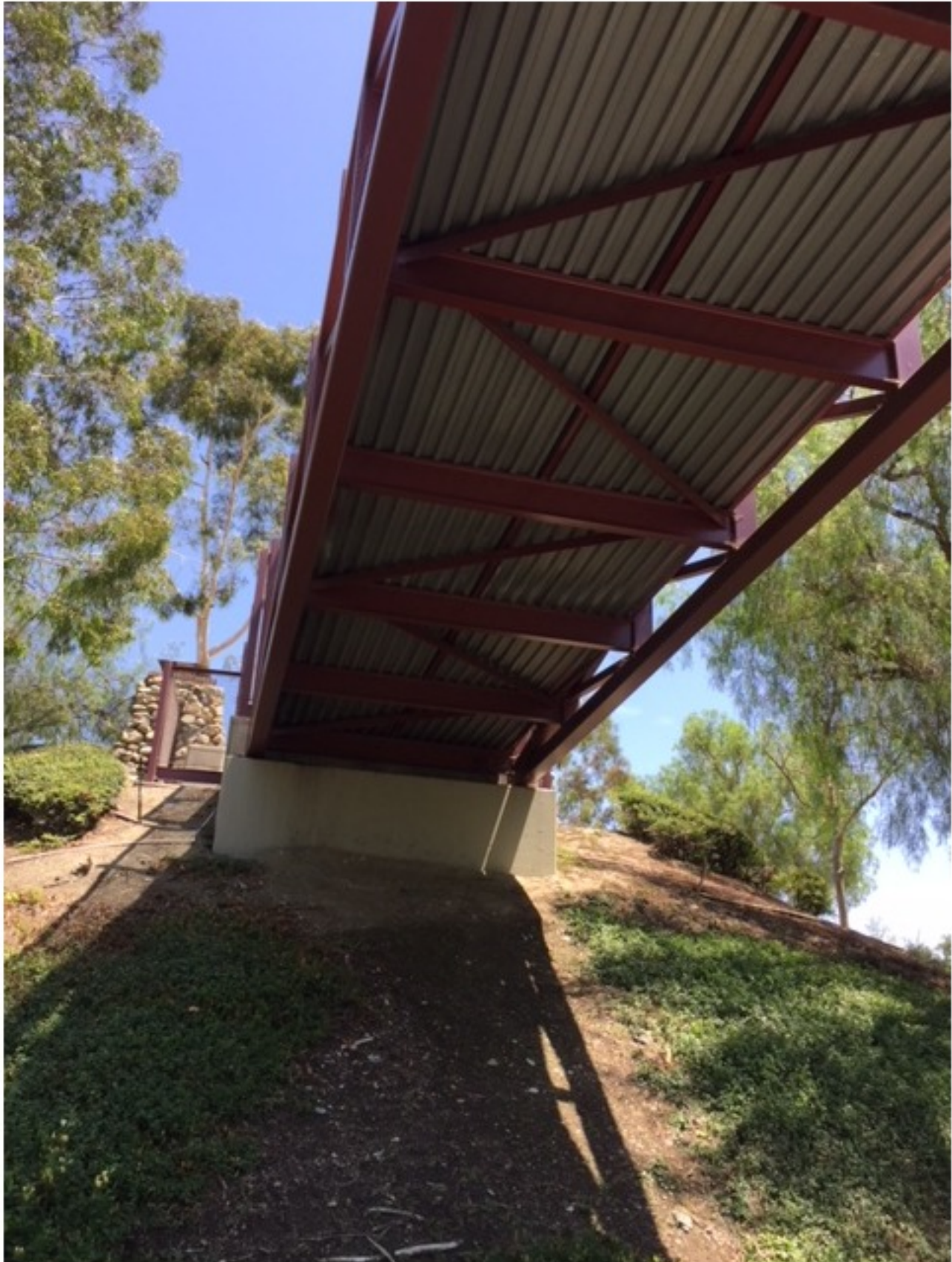
Photo No. 1 Deck soffit is covered by corrugated metal sheet
