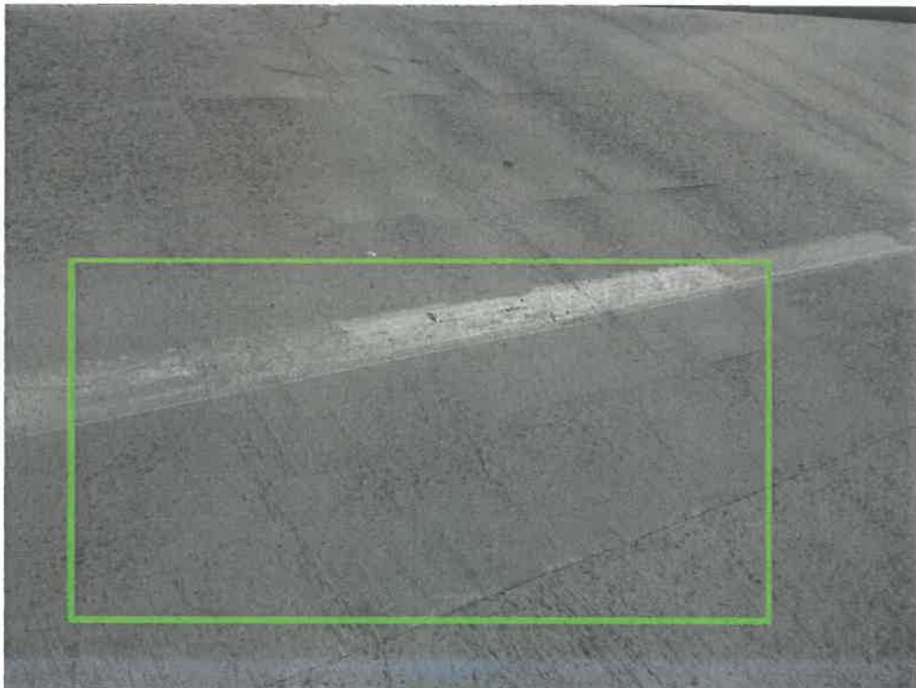
Photo No. 6 Deck transverse cracks.
