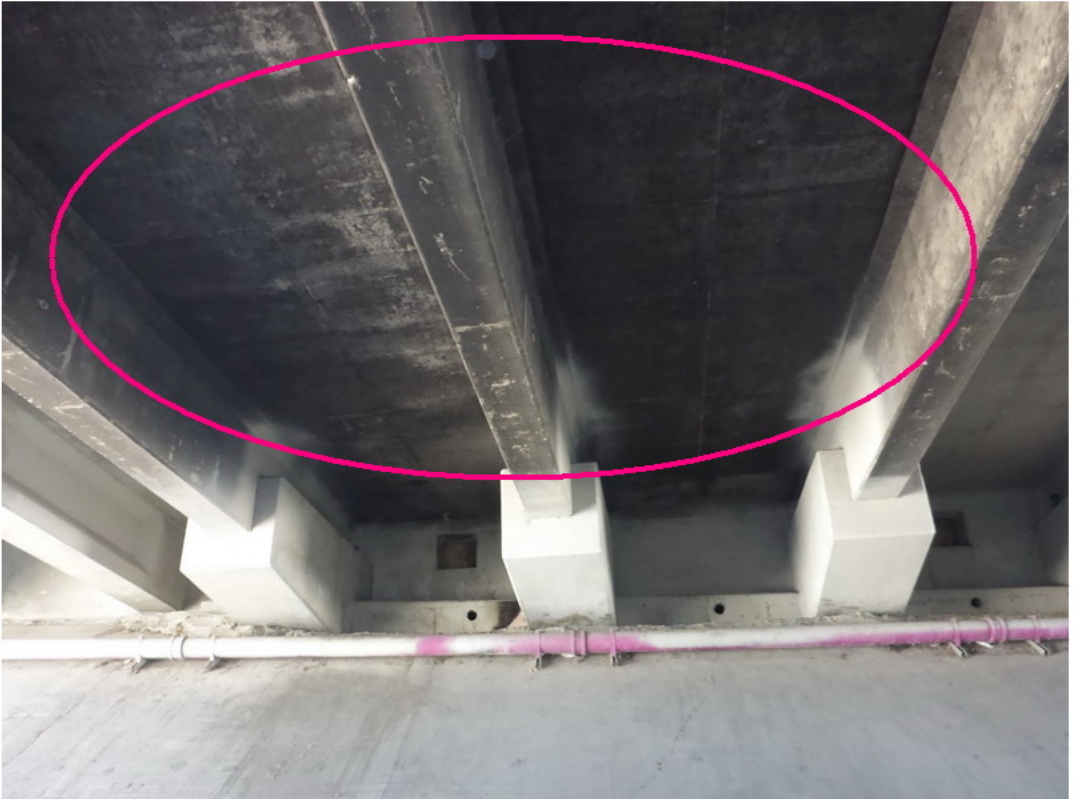
Photo No. 8 Soot is noticed at the westerly span under the RC girders.
