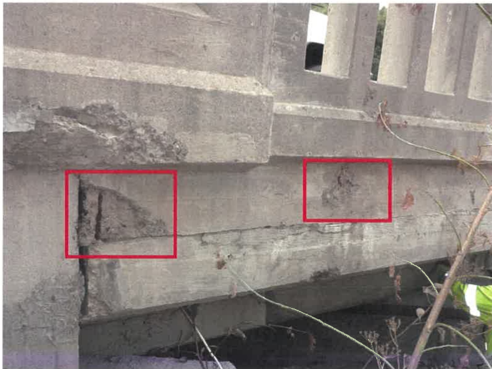
Photo No. 7 North deck elevations has 10 spalls with exposed rebars mainly in spans 2 and 3.
