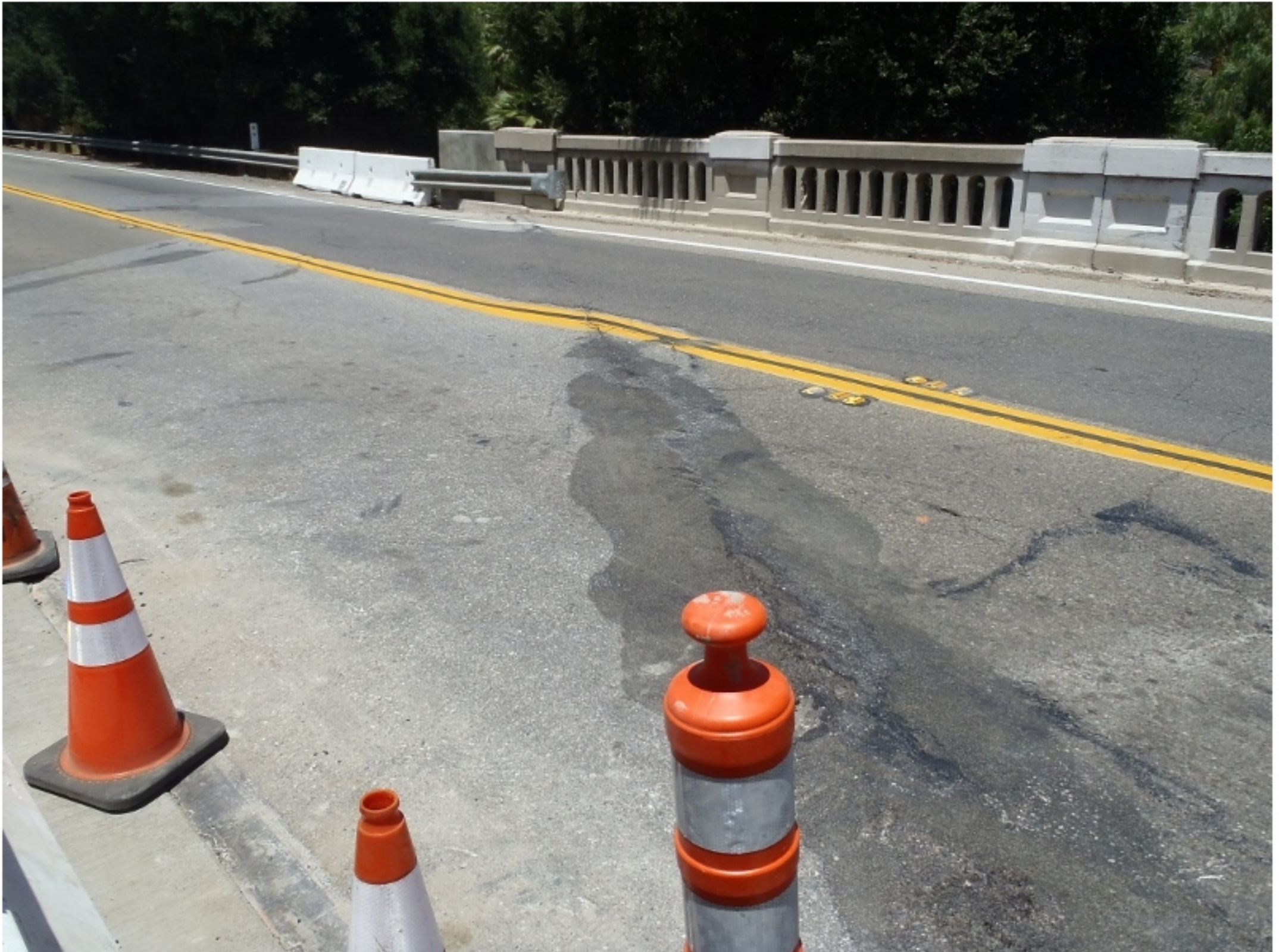
Photo No. 1 JOINT CONDITION AT WESTERN ABUTMENT
