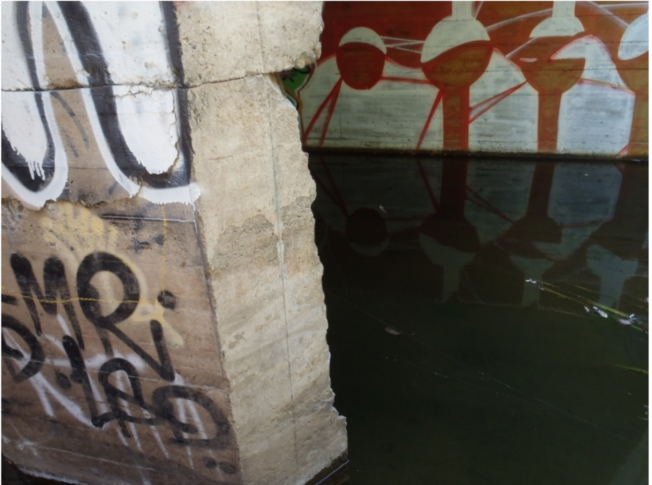
Photo No. 1 A SPALL ON THE MIDDLE PIER WALL AT WESTERN SIDE
