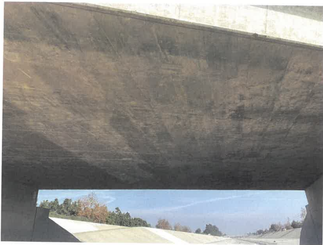
Photo No. 3 Underside View
