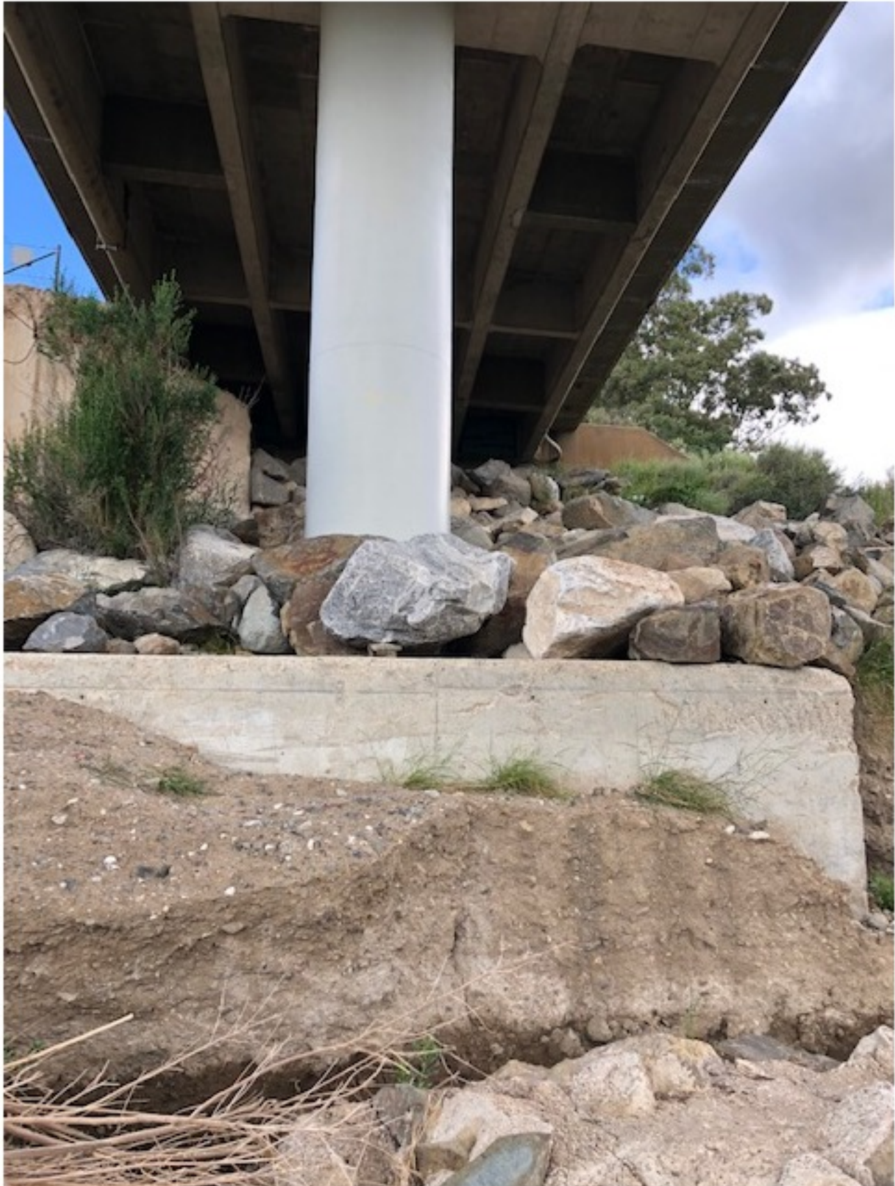
Photo No. 1 Bent #2 with a minor washout due to recent rain
