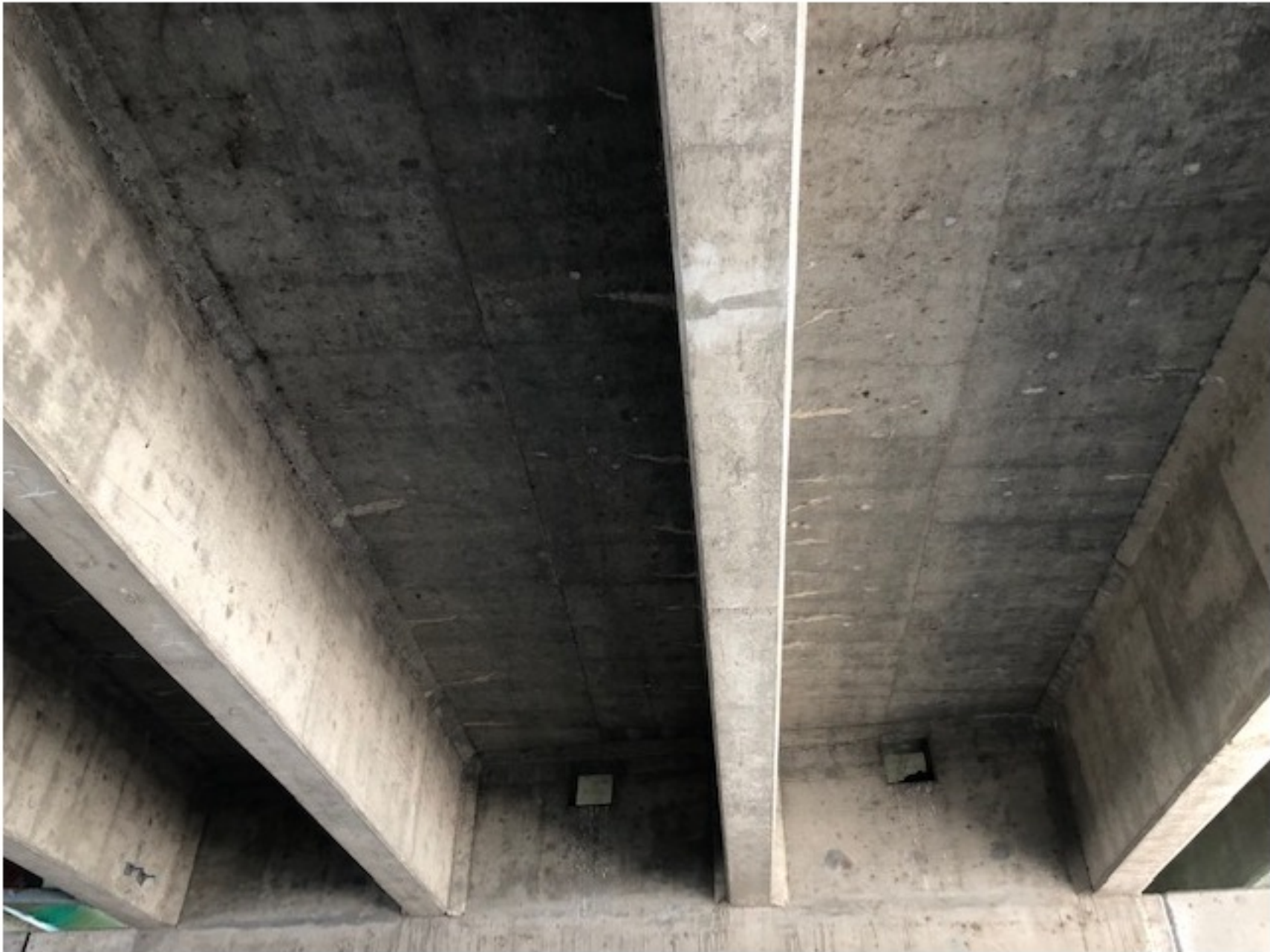
Photo No. 1 PC beam girders
