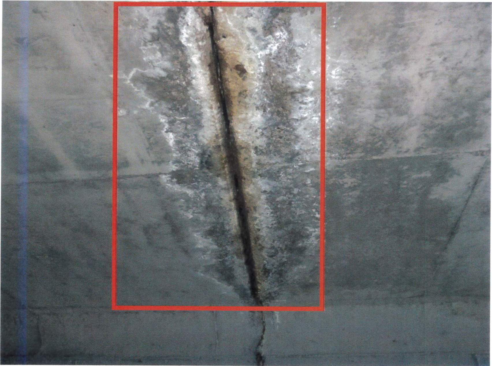
Photo No. 2 White efflorescence at the construction joint.
