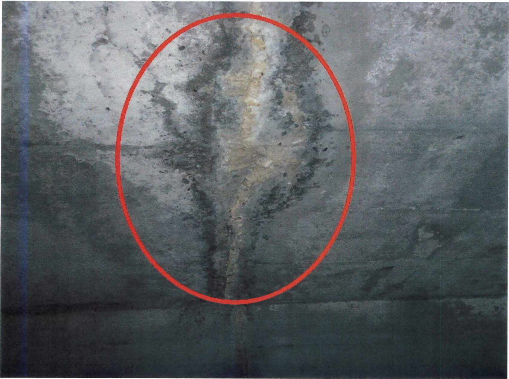
Photo No. 3 White efflorescence at the construction joint.
