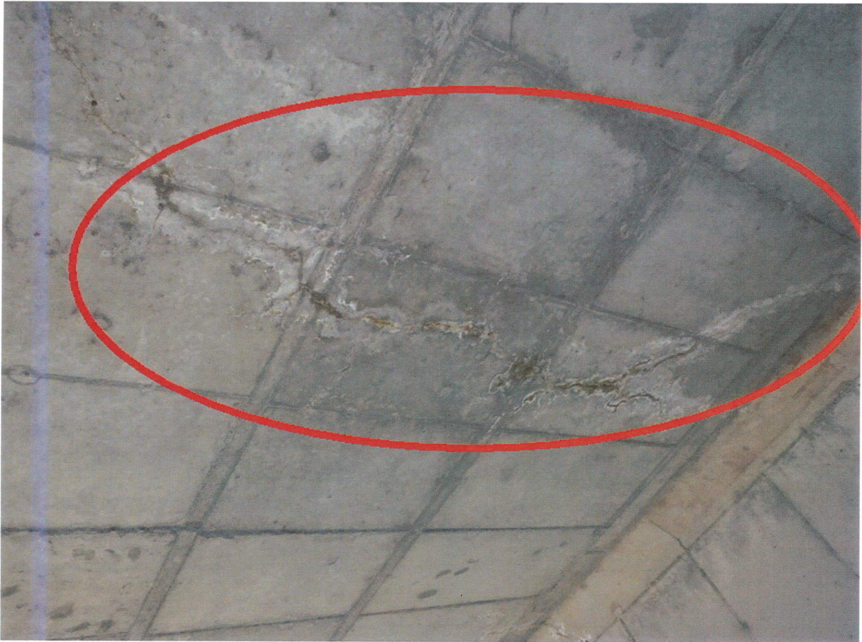
Photo No. 4 Cracks with brown efflorescence at the soffit of the culvert.
