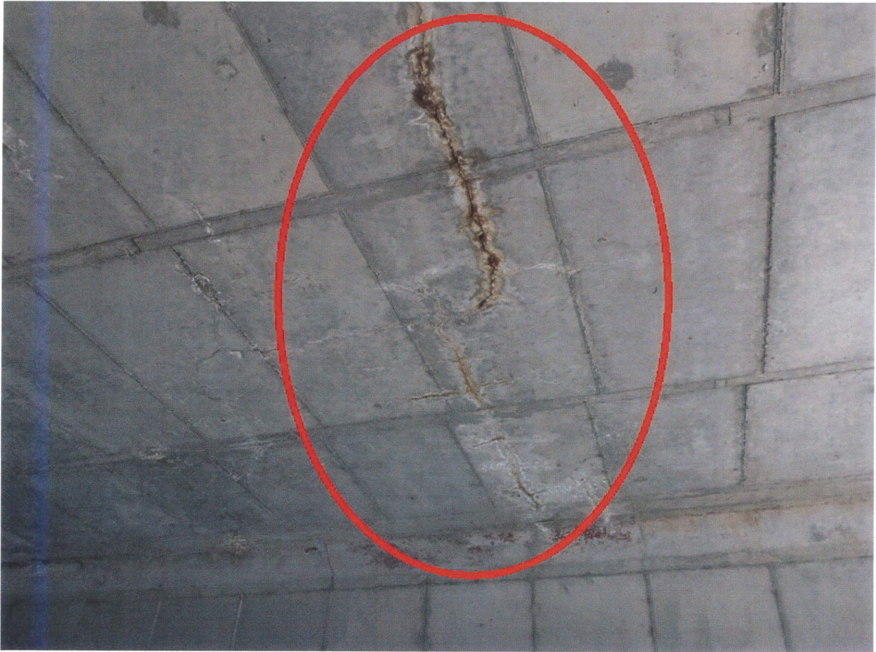
Photo No. 5 Cracks with brown efflorescence at the soffit of the culvert.
