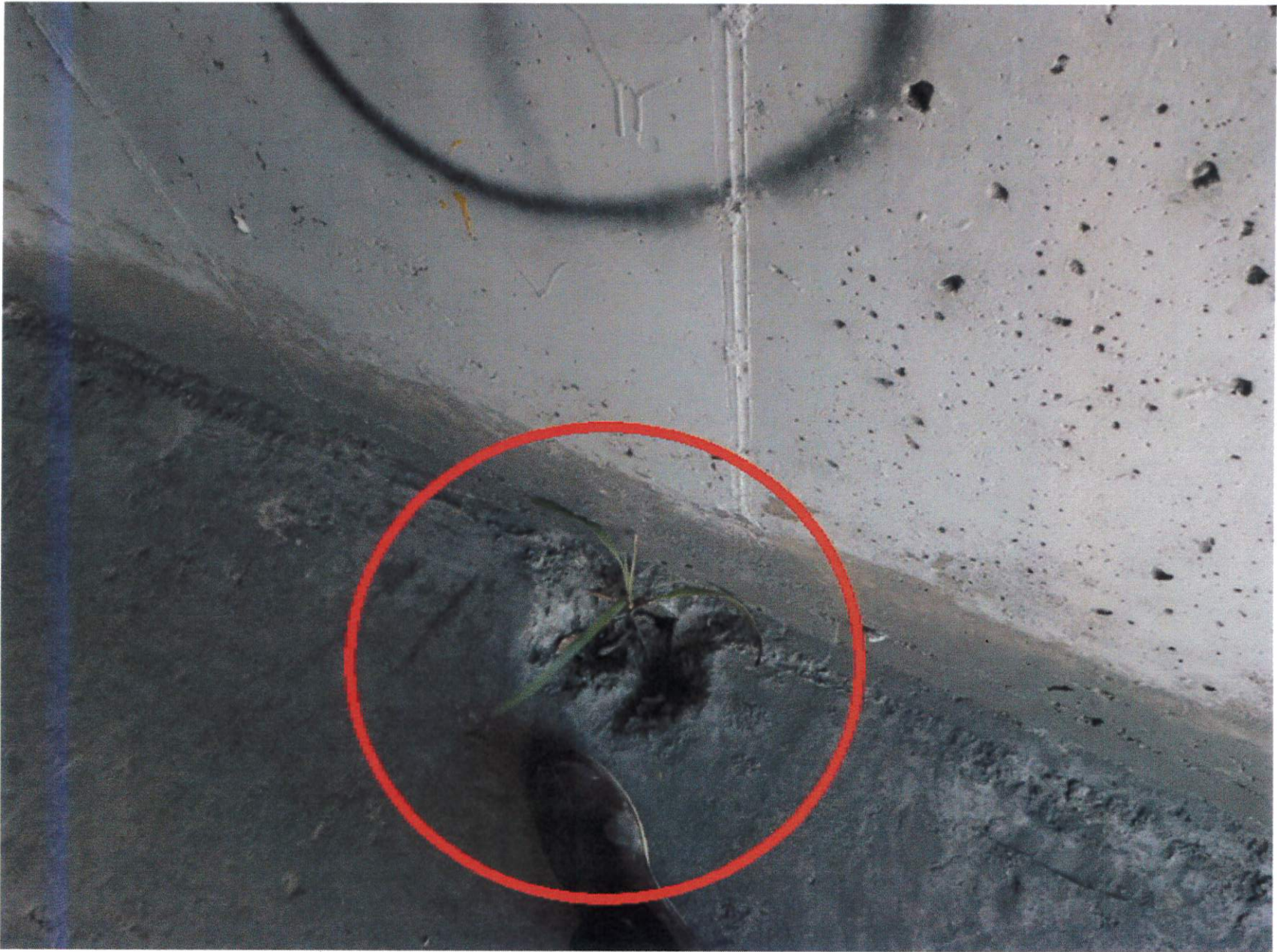
Photo No. 8 Spall at the invert of barrel 2 at 15 feet from west end.
