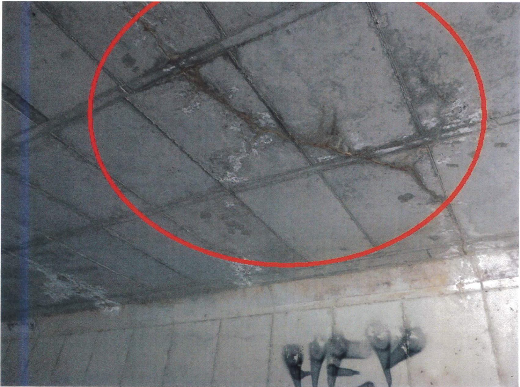
Photo No. 3 Cracks with brown efflorescence at the soffit of the culvert.
