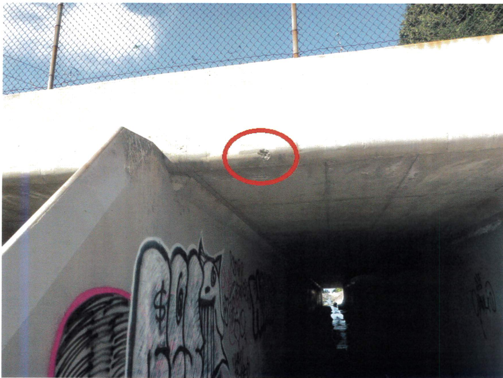
Photo No. 3 Spall at the east end of barrel 2.
