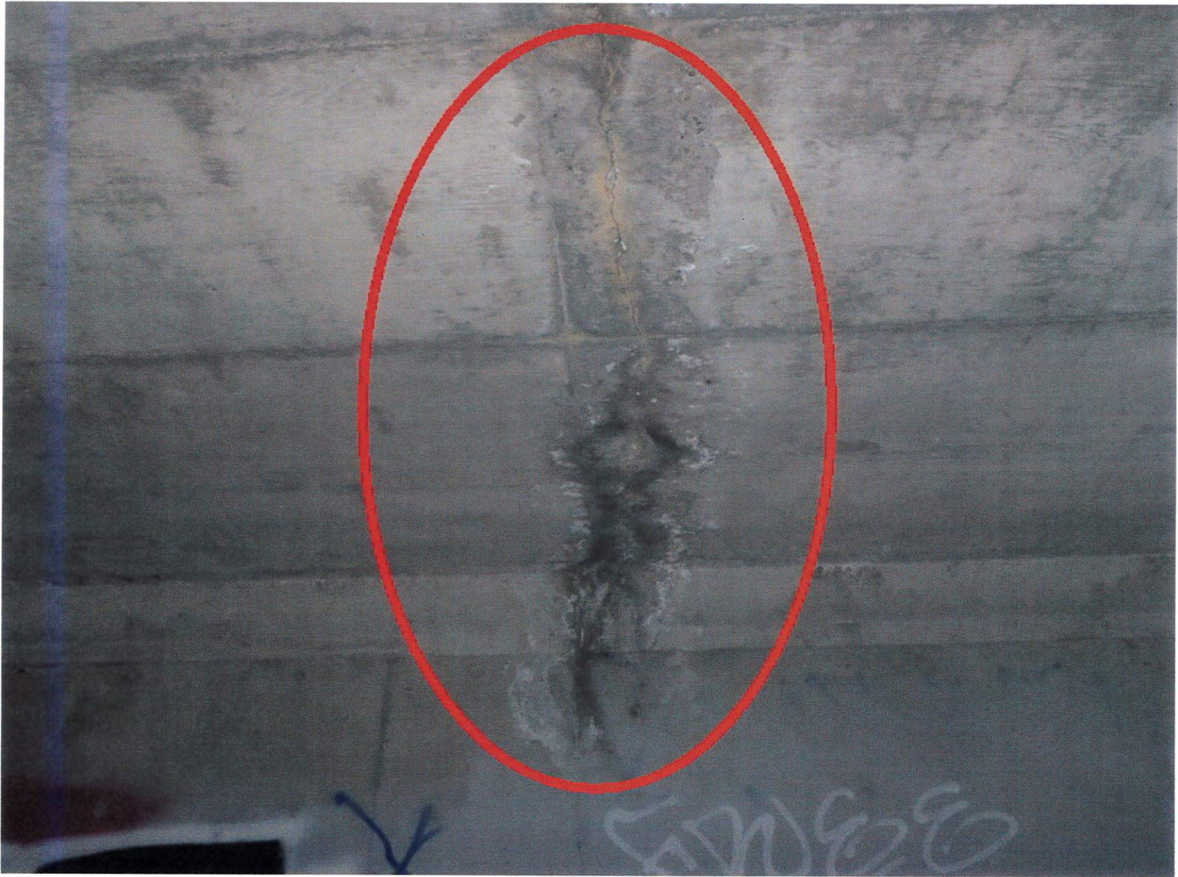
Photo No. 2 Soffit cracks 0.08 inches wide with efflorescence.
